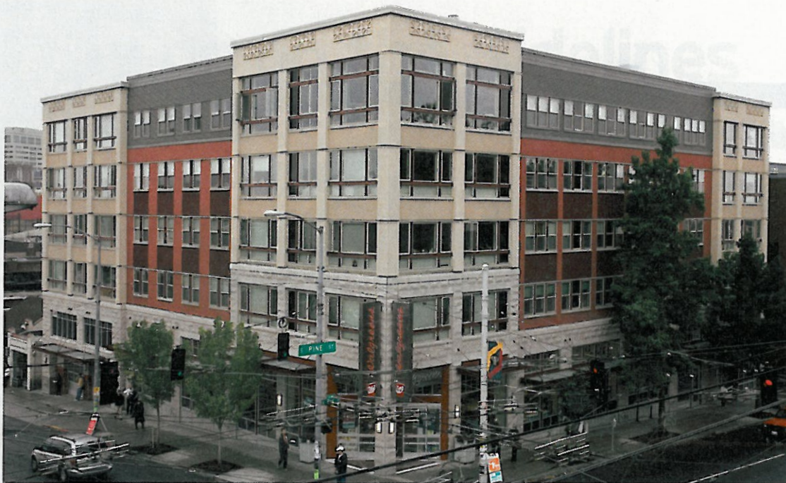
Transit-oriented and energy-efficient, Broadway Crossing has room to become even more sustainable by producing its own energy. The roof is wired for solar panels, and the developer is actively pursuing grant opportunities. (Photo by Tim Matsui)
